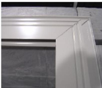
The encapsulation should hang off the pool wall 1/2" – 5/8" so that the tile will be flush with the front side of the encapsulation. If the gunite walls are slightly out of square you may have this overhang vary so that after brown coat and tile the pool (and cover tracks) will be a true rectangle.
